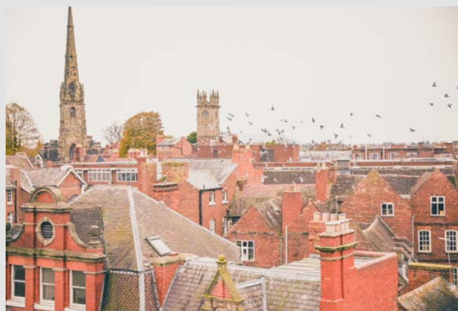
Figure 12 View of Shrewsbury's roofscape with St Alkmund's Church spire and St Julian tower.
