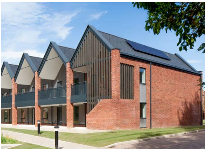
Figure 73 Orientating roofs to incorporate PVs. Radbrook Village, Shrewsbury. Photo credit AHR Architects.
