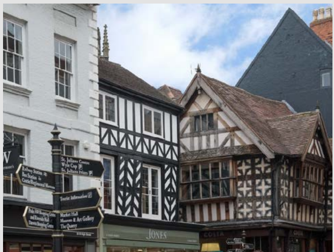
Figure 10 Variety of buildings along High Street.
