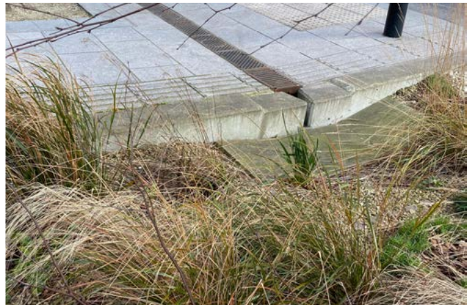
Figure 43 Sustainable Urban Drainage including rain gardens, within the design of public realm.
