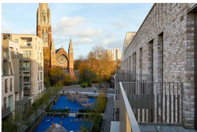
Figure 72 Balconies can project up to 2m and should be fully integrated in the design of the building.
